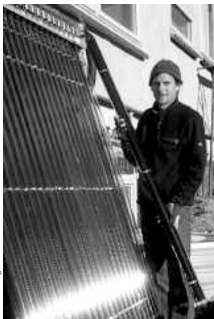
Wyoming Outdoor Council board president, Scott Kane, installing a solar panel.
